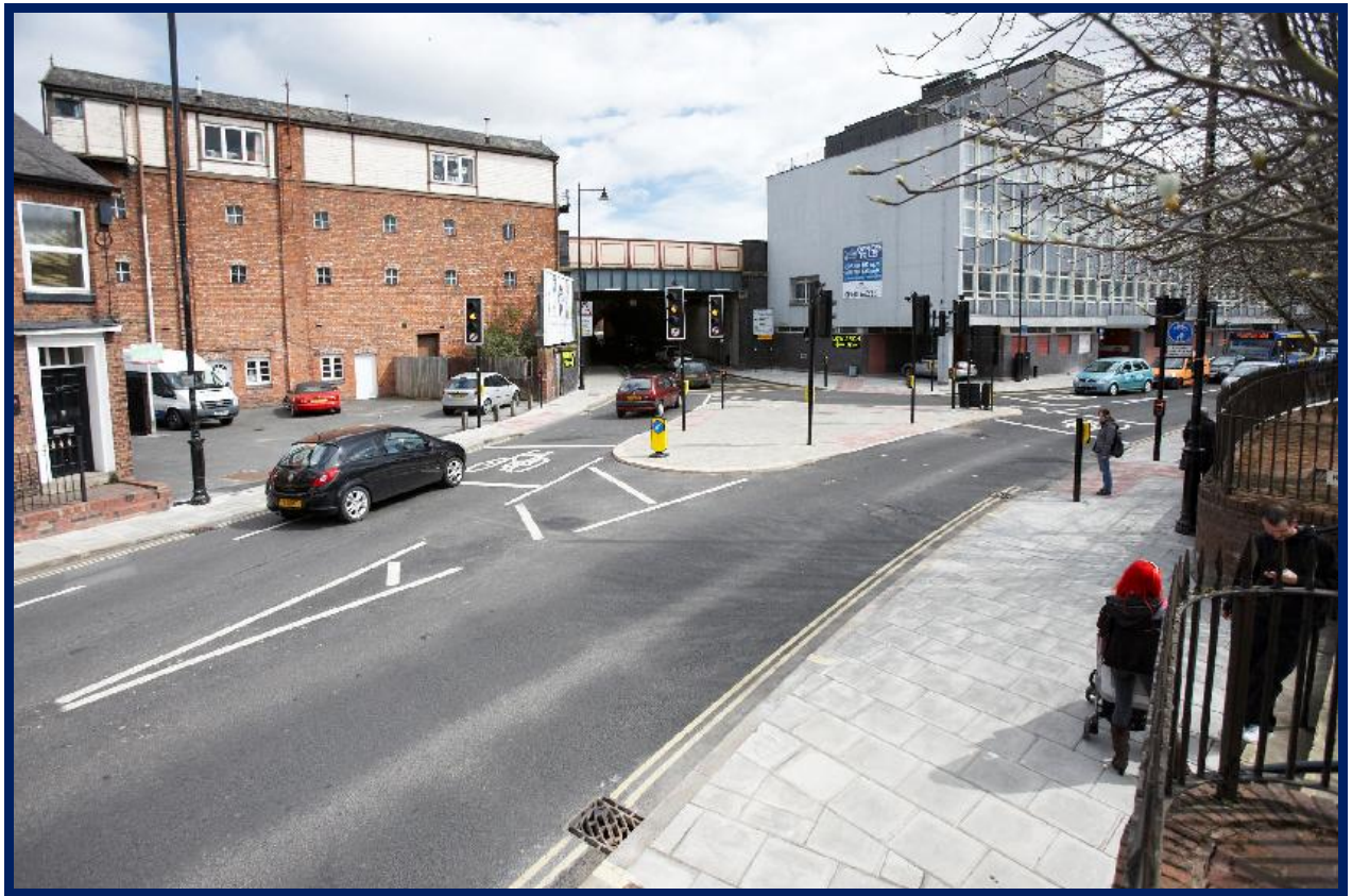
Chester Street Road Improvements
